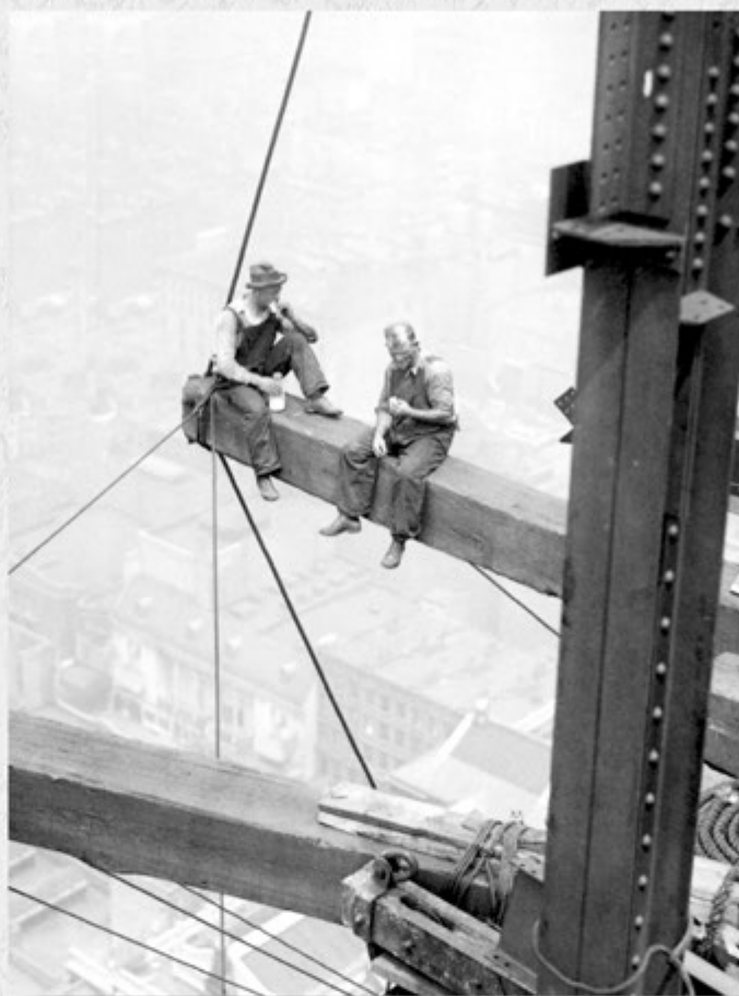
ANONIMO Workers sitting on steel beam
